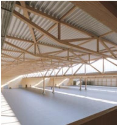
As a screw specialist for timber construction, sustainability and environmental protection are key components for the growth strategy of **SWG Schraubenwerk Gaisbach GmbH - Produktion**. The company's own production floor with offices demonstrates that it is possible to construct industrial buildings out of wood instead of steel and reinforced concrete, while capturing eleven times more CO<sub>2</sub> than conventional buildings.
