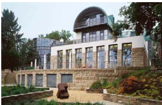
> Würth Haus Berlin, one of the two representative offices of the Würth Group
